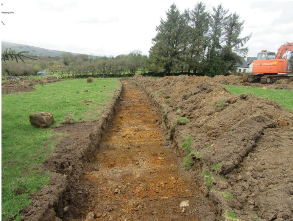
Plate 6 - Test Trench 10 – After excavation
