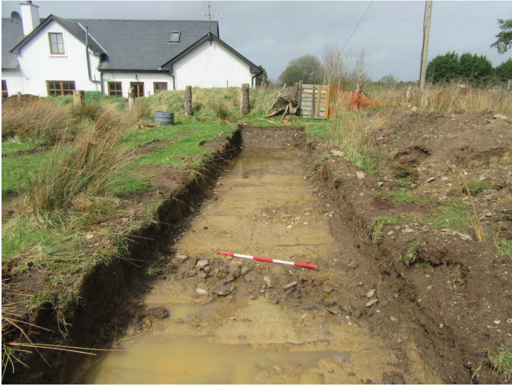
Plate 5 - Land drain in Test Trench 5
