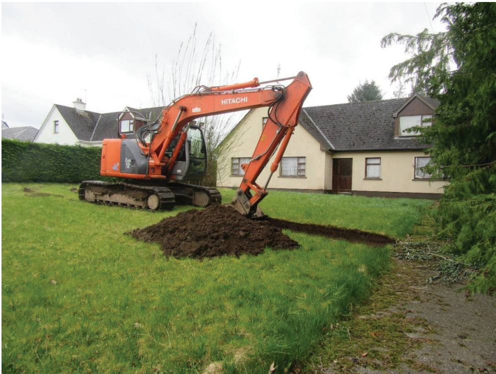
Plate 10 -Test Trench 1 - in front garden of existing house on proposed development site
