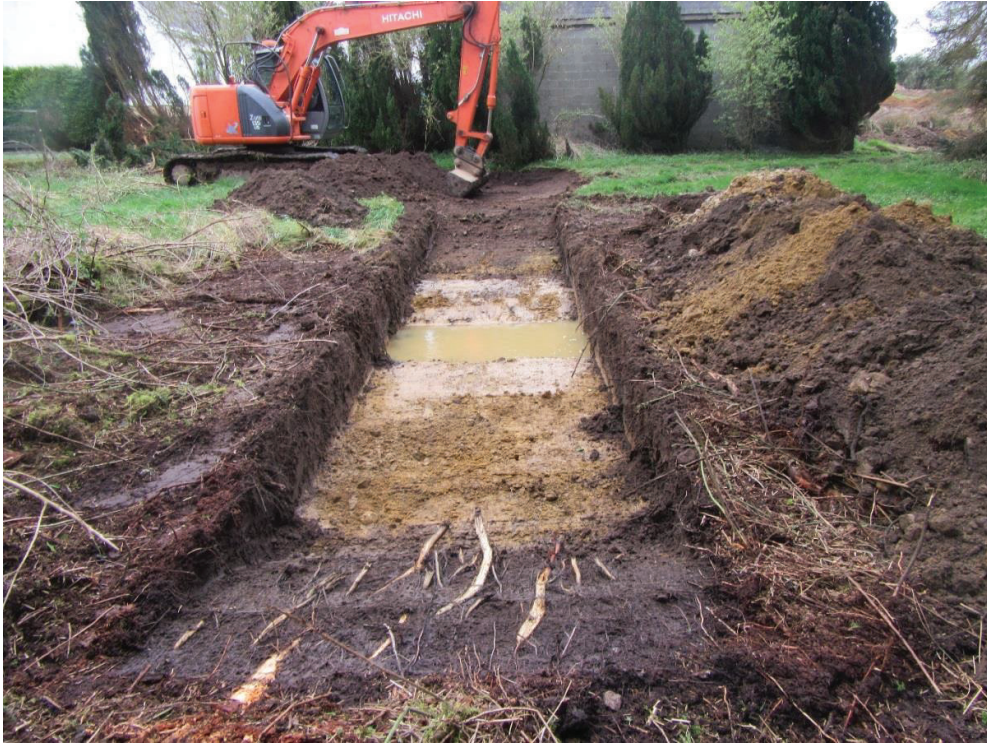
Plate 9 - Test Trench 2 - at rear of existing house on proposed development site
