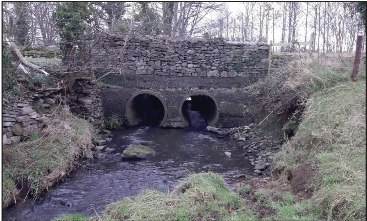
Figure 2.5 View of bridge no. 2 (facing upstream) 20 th Jan 2020.
