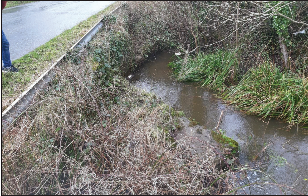
Figure 2.4 View of bridge no. 1 (facing downstream) 21 st Feb 2020.
