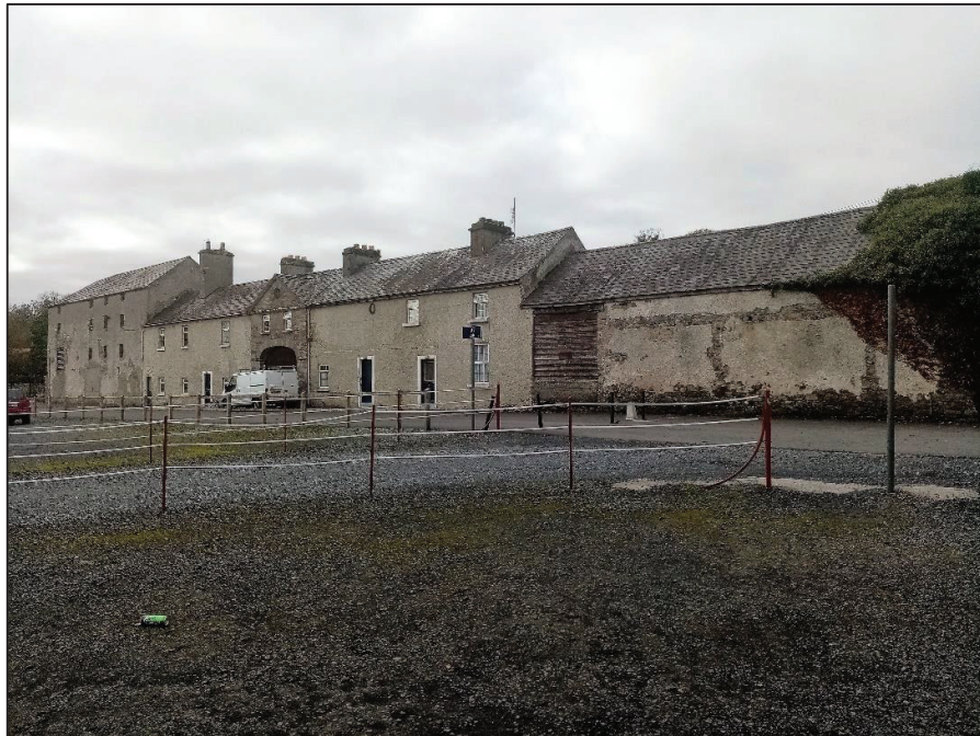
Plate 2 Part of the Farm Complex (Reg No. 31308801) associated with Westport House
