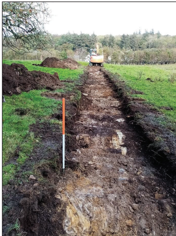
Plate 8 Shallow clay above limestone rock and marl Test Trench 6
