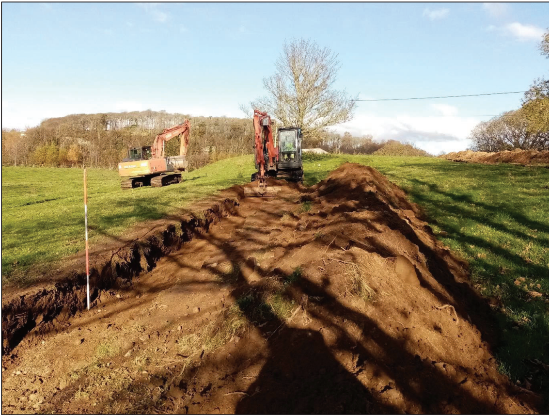
Plate 21 Looking north-east along line of Test Trench 22 with 21 to right of picture. Grassy rise behind diggers represents edge of quarry
