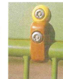
IMAGE 05: SPECIAL VANDAL FIXINGS WITH STAINLESS BOLTING OR SIMILAR APPROVED / EQUIVALENT ASSEMBLY
