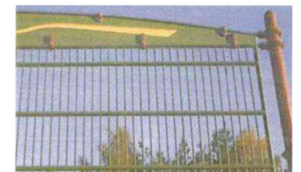
IMAGE 04: PANEL EXTREMELY RIGID WITH STEEL FRAME AND 10MM BARS OR SIMILAR APPROVED / EQUIVALENT ASSEMBLY UNIT
