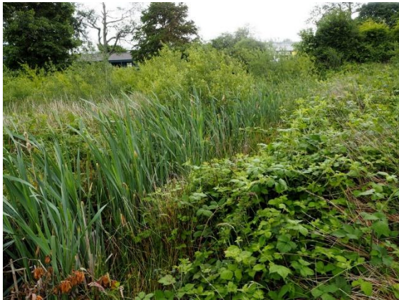
Drain between section 3 and 4
