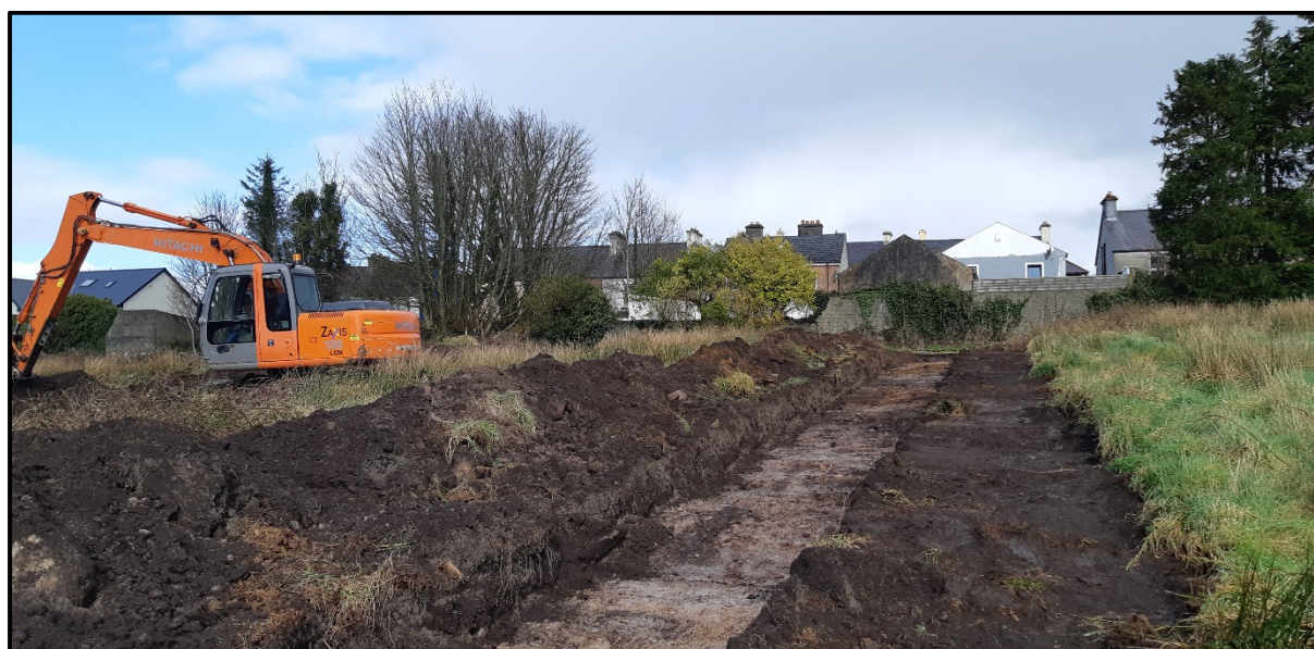
Plate 5 Looking north to general view of Test Trench 11.
