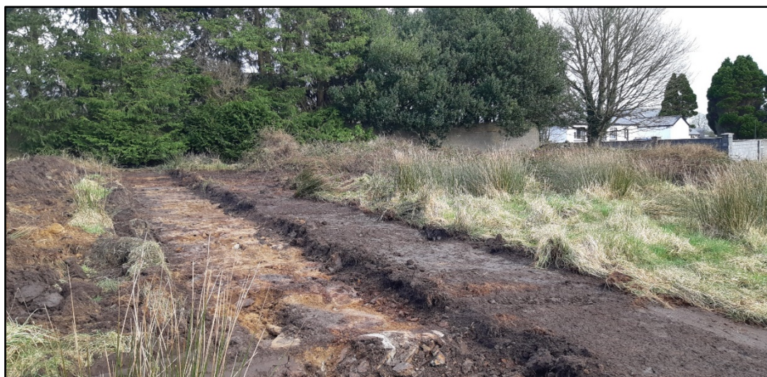
Plate 4 Looking north-east to Test Trench 10. Rock coming through boulder clay (C8) in foreground.
