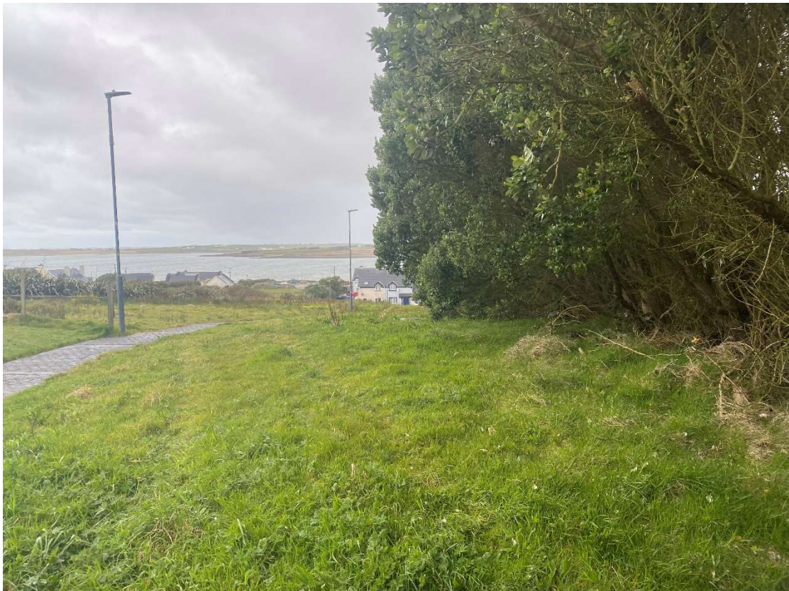
Photo 2. Existing street lighting on the site.
