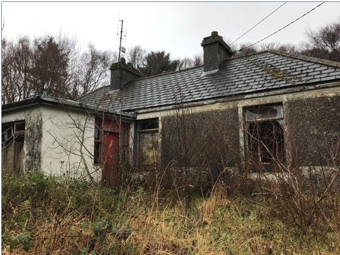
Plate 2-4 A derelict house with surrounding agricultural sheds occurs within the centre of the site and is classified as Buildings and Artificial Surfaces (BL3).
