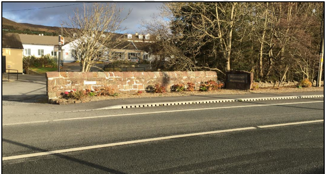
Figure 2.4 Single span concrete bridge (bridge no.1)
