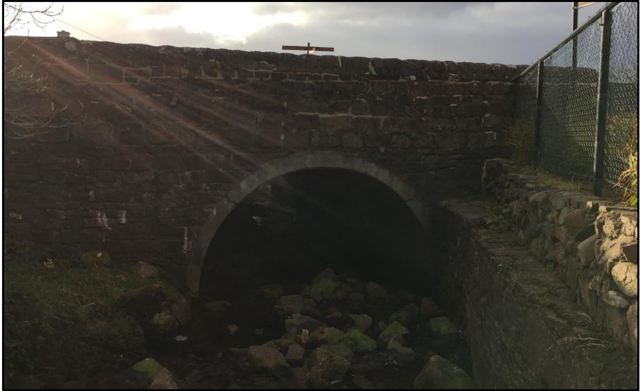
Figure 2.5 Concrete culvert (bridge no.1)
