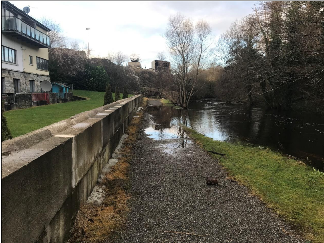
Plate 2-1 River Carrowbeg, view downstream, with adjacent Cois Abhainn housing estate.
