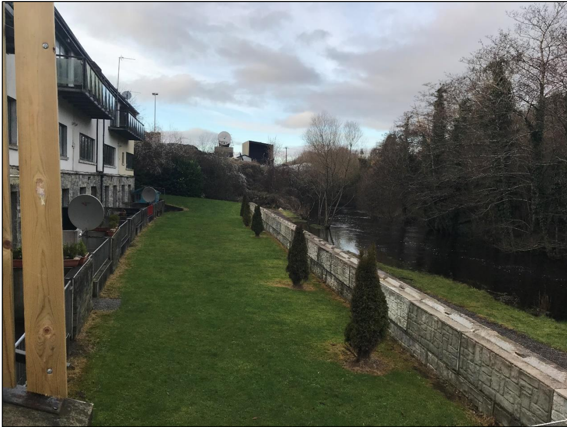
Plate 2-4 The proposed flood defence wall will occur on the lawn between the existing flood defence wall and the Cois Abhainn housing estate, classified as amenity grassland
