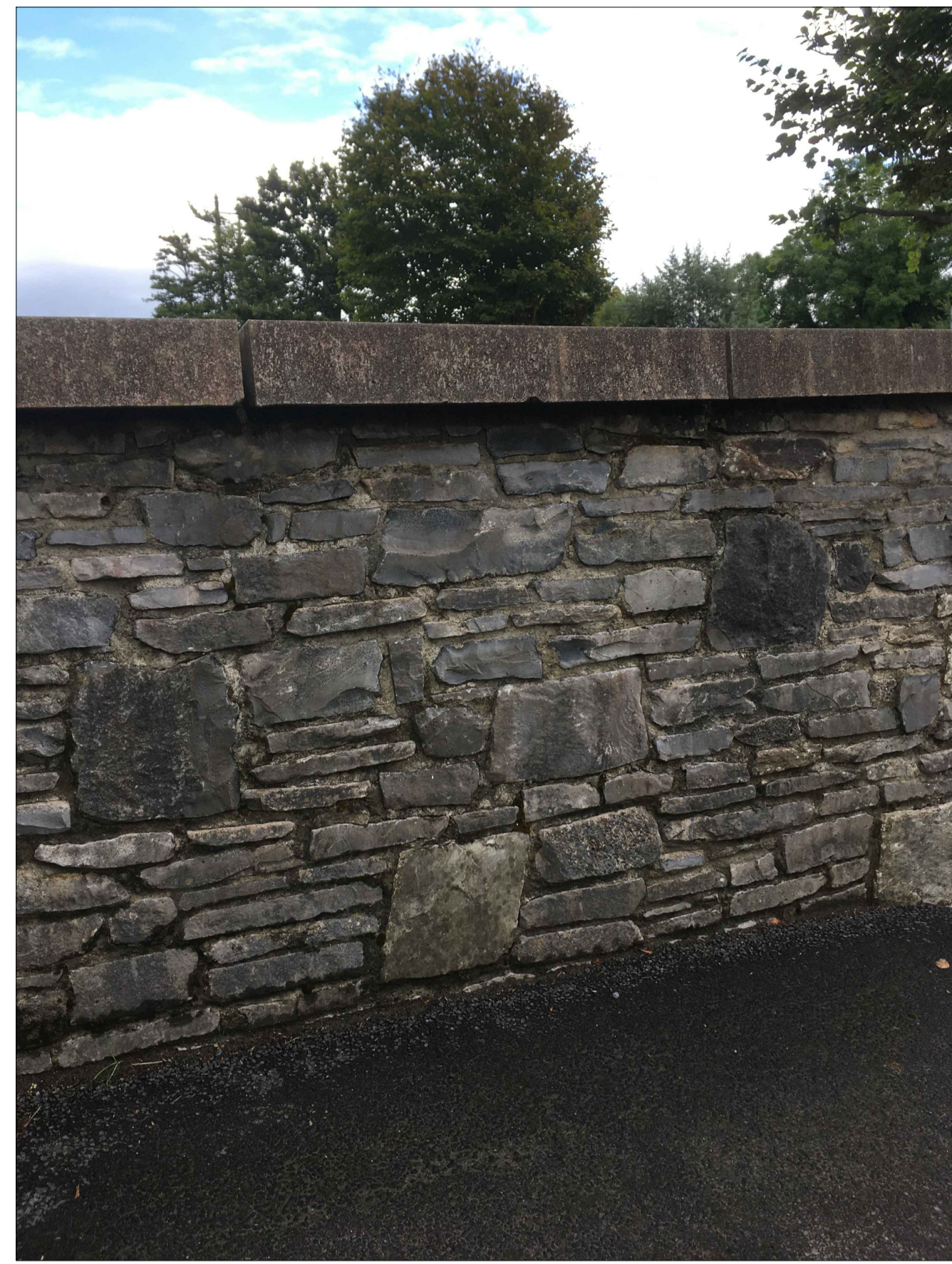
PROPOSED FLOODWALL FINISH [NATURAL STONE CLADDING]
