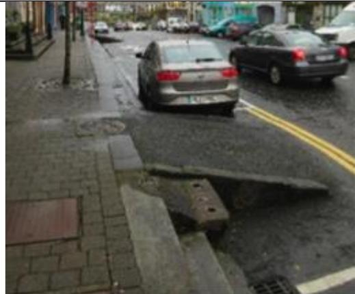
The existing ramped access will be retained in this location but upgraded to comply with existing disability access requirements at the proposed road crossing. There will be no further loss of historic stone .
