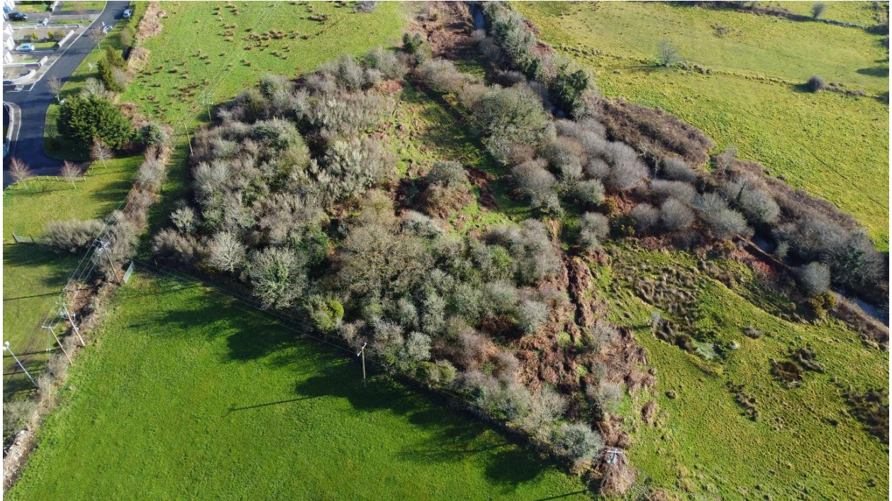
Figure 10: Looking North: Ringfort-Rath MA063-005 Lowpark Townland, Charlestown (Drone Image John Gallagher MCC 2022)
