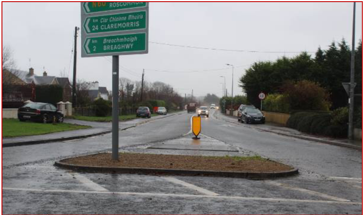
Figure 6.9: Parking within N60 Verges and Footpaths adjacent to Kilkenny Cross Roundabout
