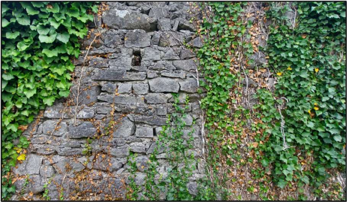
Plate 3.5 Stone wall habitat (BL1) at the north end of the site
