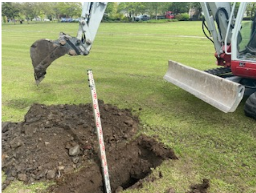
Trial Hole No 5 – 1200mm depth to bearing ground
