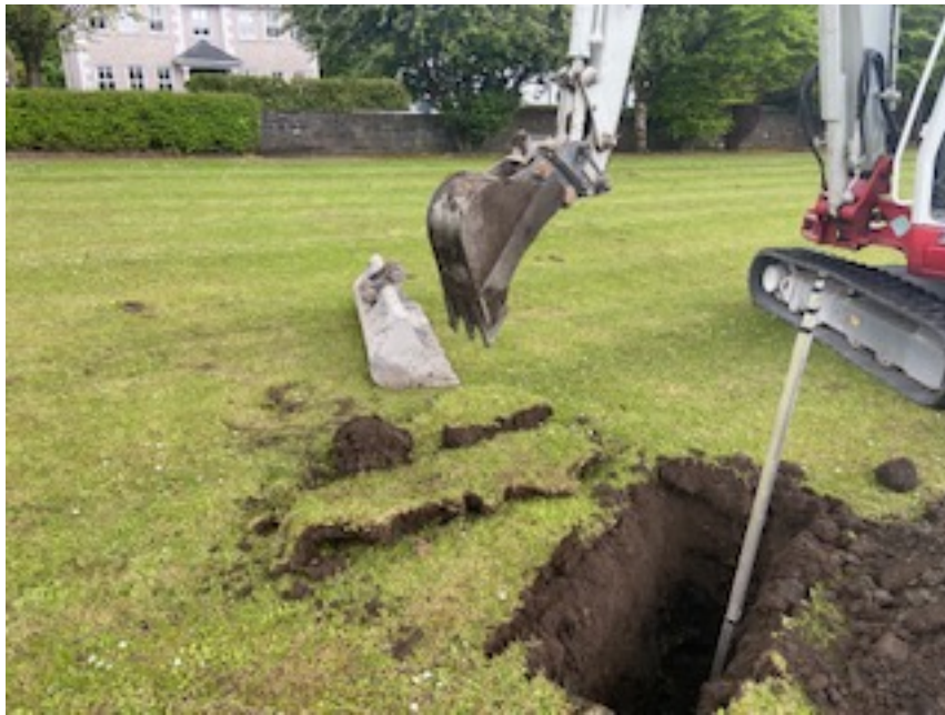
Trial Hole No 3 – 1200mm to bearing ground
