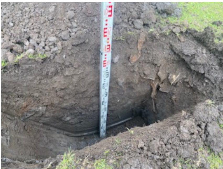
Trial Hole No 1 – 1200mm depth to bearing ground
