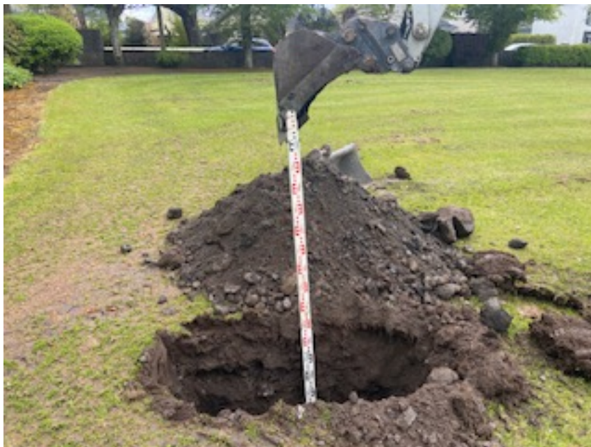
Trial Hole No 4 – 1200mm to bearing ground
