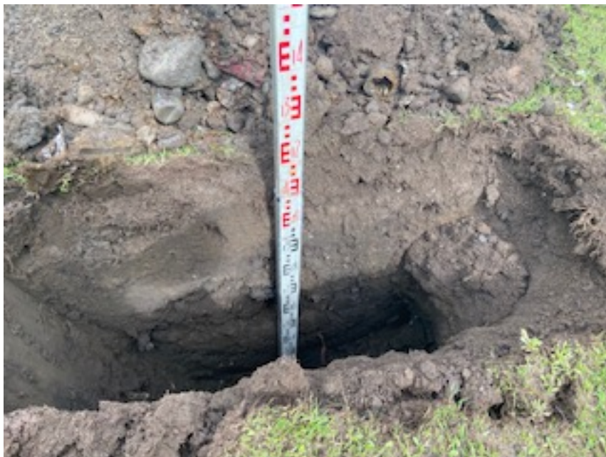
Trial Hole No 5 – Clay/Waste material mix to 1000mm below surface
