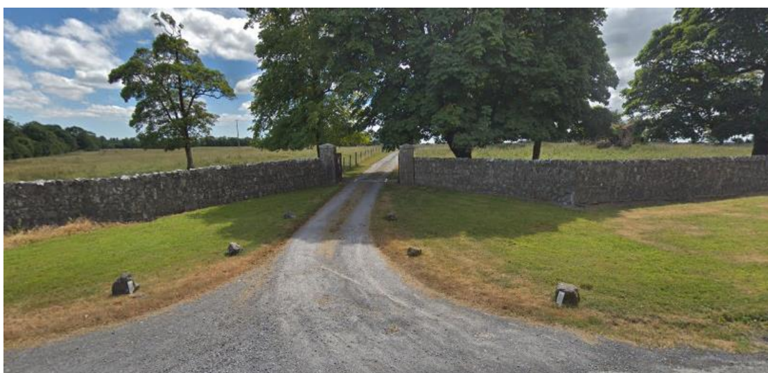
Figure 2-7 Boundary wall and entrance to Cloghans House (RPS, 2065)
