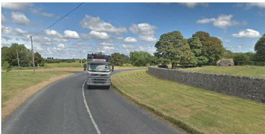
Figure 2-1 Existing poor alignment along the R332 Regional Road
