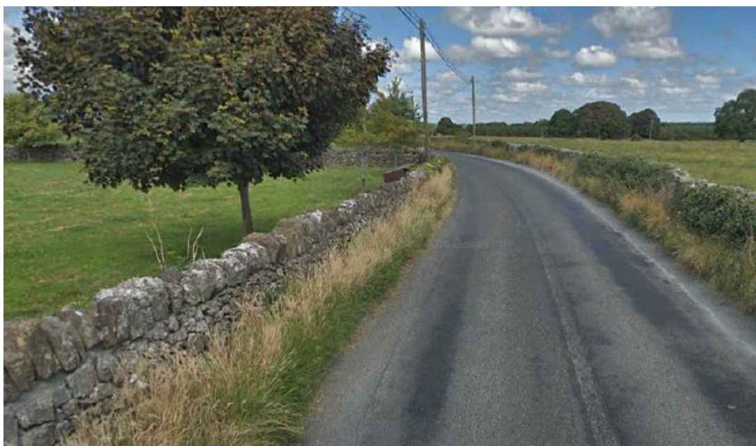
Figure 2-2 Existing poor alignment along the R332 Regional Road
