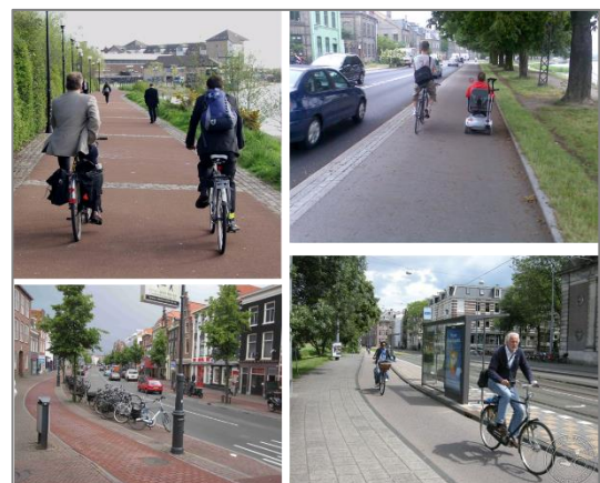
Figure 7-4: Indicative layouts for segregated cycle tracks
