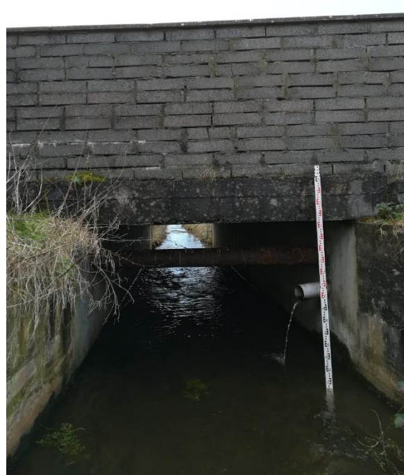
Figure 2.5 Downstream Bridge No.1 on western site boundary (facing downstream)
