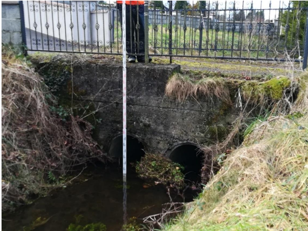
Figure 2.6 Downstream Bridge No.2 (facing downstream)
