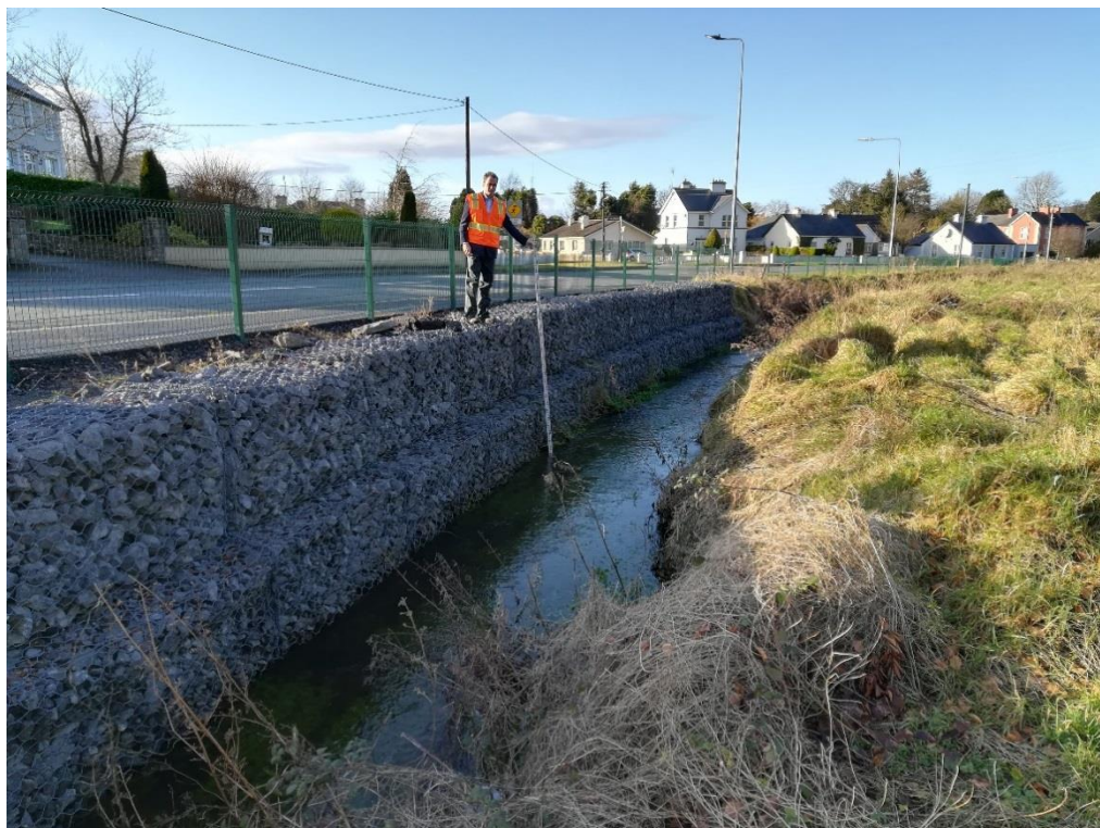
Figure 2.7 Erosion protection downstream (facing downstream)
