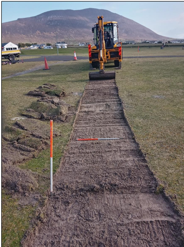
Plate 1 De-sodding Test Trench 1 looking North with Keel Caravan Park in the background
