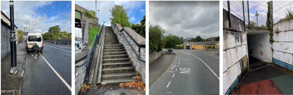
Figure 7-15 – Absent connections between the Greenway and the town centre on Altamont Street
