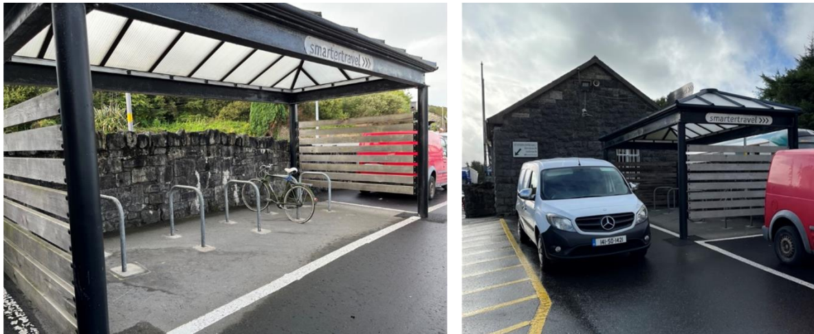
Figure 7-17 – Cycle parking at Westport Station
