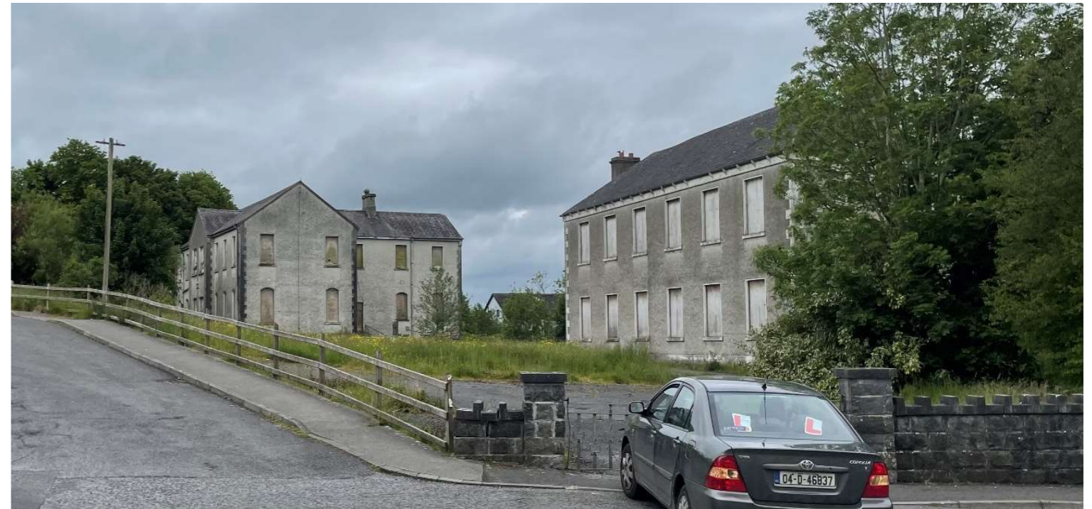
View of Former School from Bridge Street (Current State)
