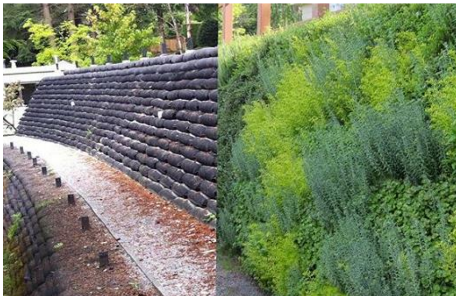
Figure 7 Pre-seeded retained slope face as constructed (left) and once established (right)
