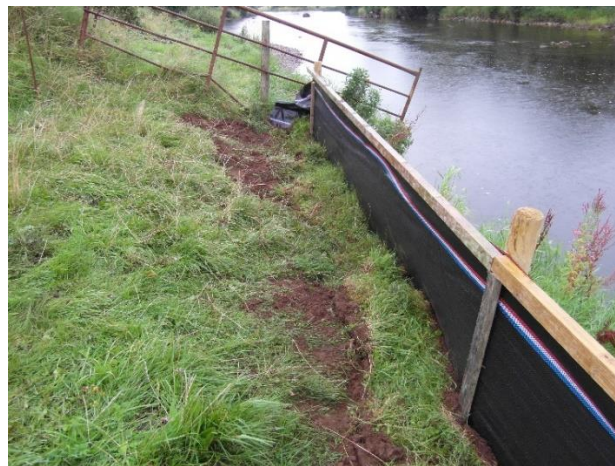
Photographs showing examples of silt fence along river bank
