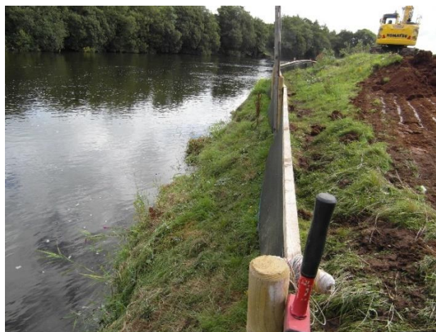
Photographs showing examples of silt fence along river bank
