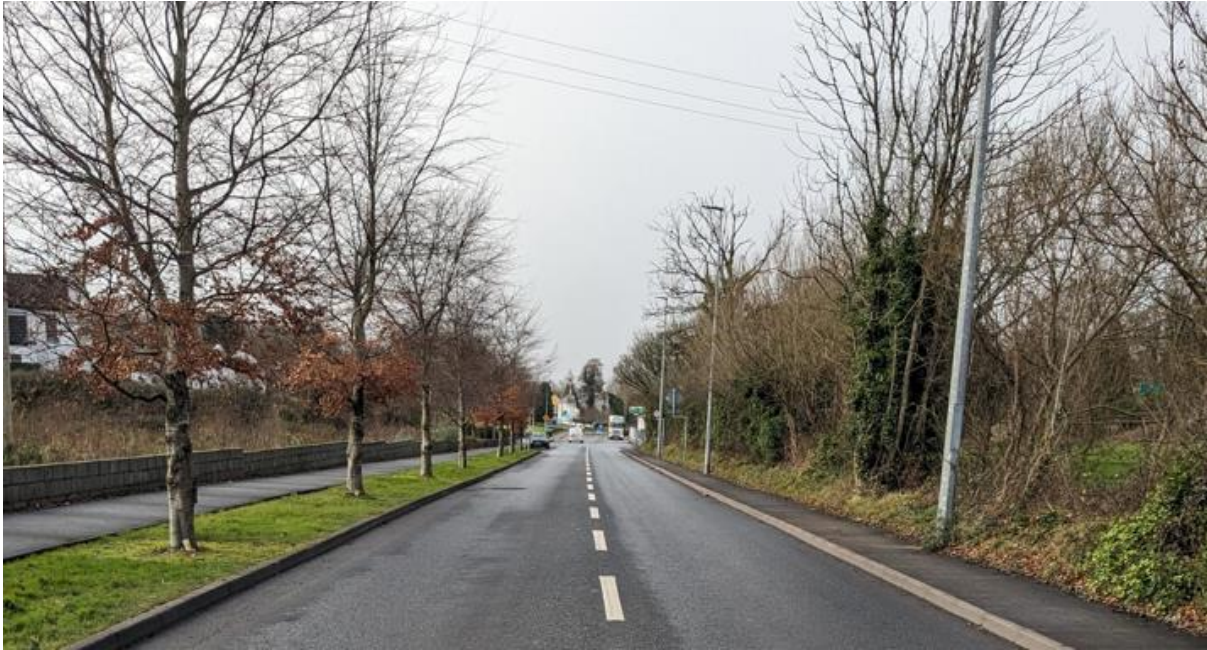
Figure 6-13: Behy Road (Westbound Direction)
