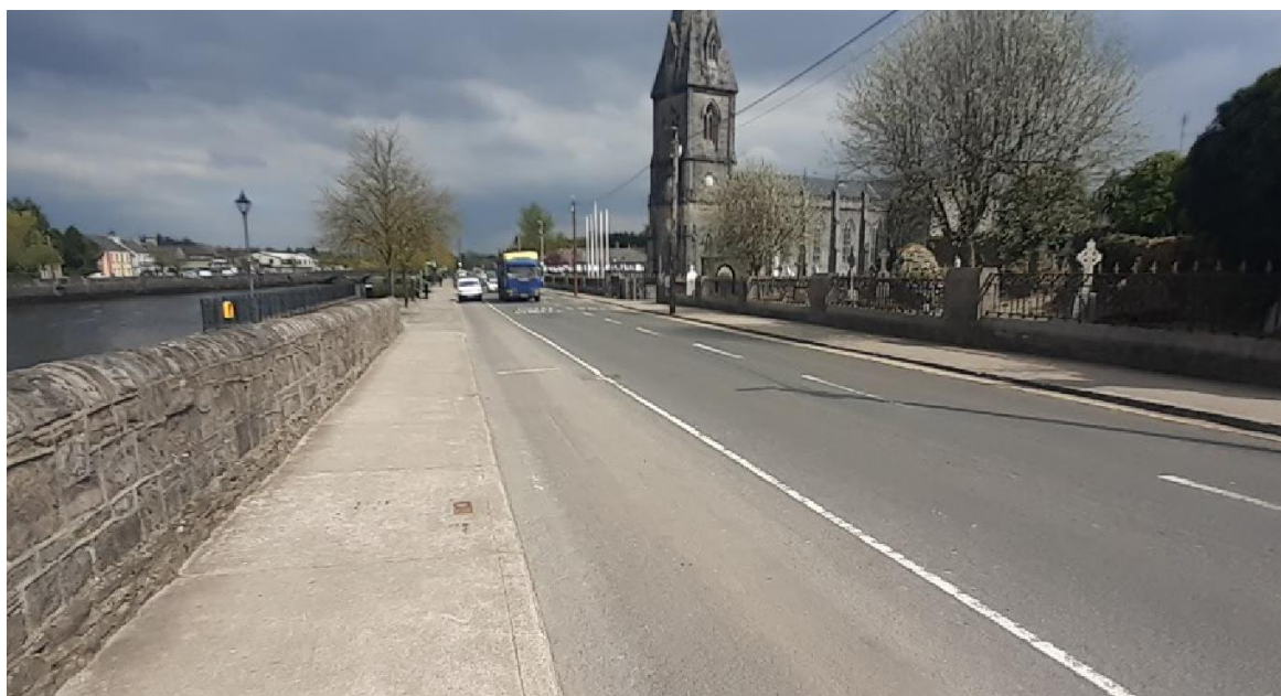
Figure 6-8: N59 Cathedral Road (Northbound Direction)
